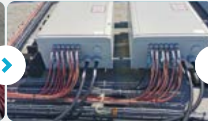
A combiner box that brings the cables together into one thick DC cable
